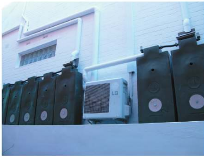
HOG fit snugly down the side passage and the threaded connections allow plumber to space the modules around the wall mounted utility boxes
