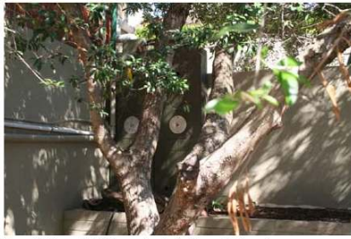
Two vertically mounted HOGs supply water for the small side garden.
